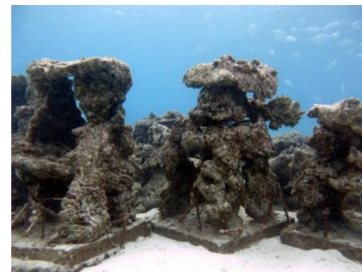
Fish habitat modules designed and fabricated by Apo Island dive rangers and fisherfolks made of rocks and cement. Photo: A. Maypa
